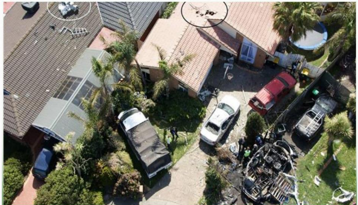
Acetylene cylinder-related damage
