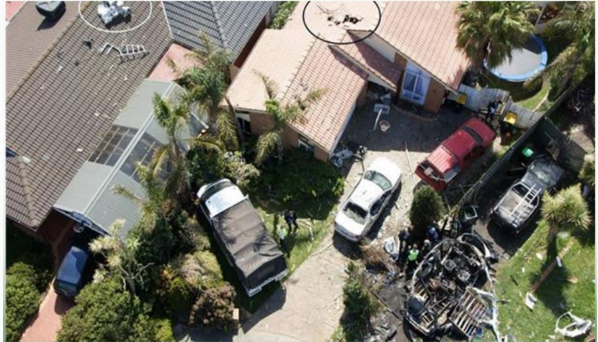
Acetylene cylinder-related damage
